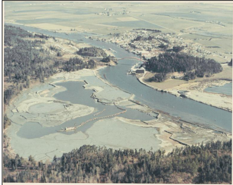
Dredging the marina and waterfront lots.
